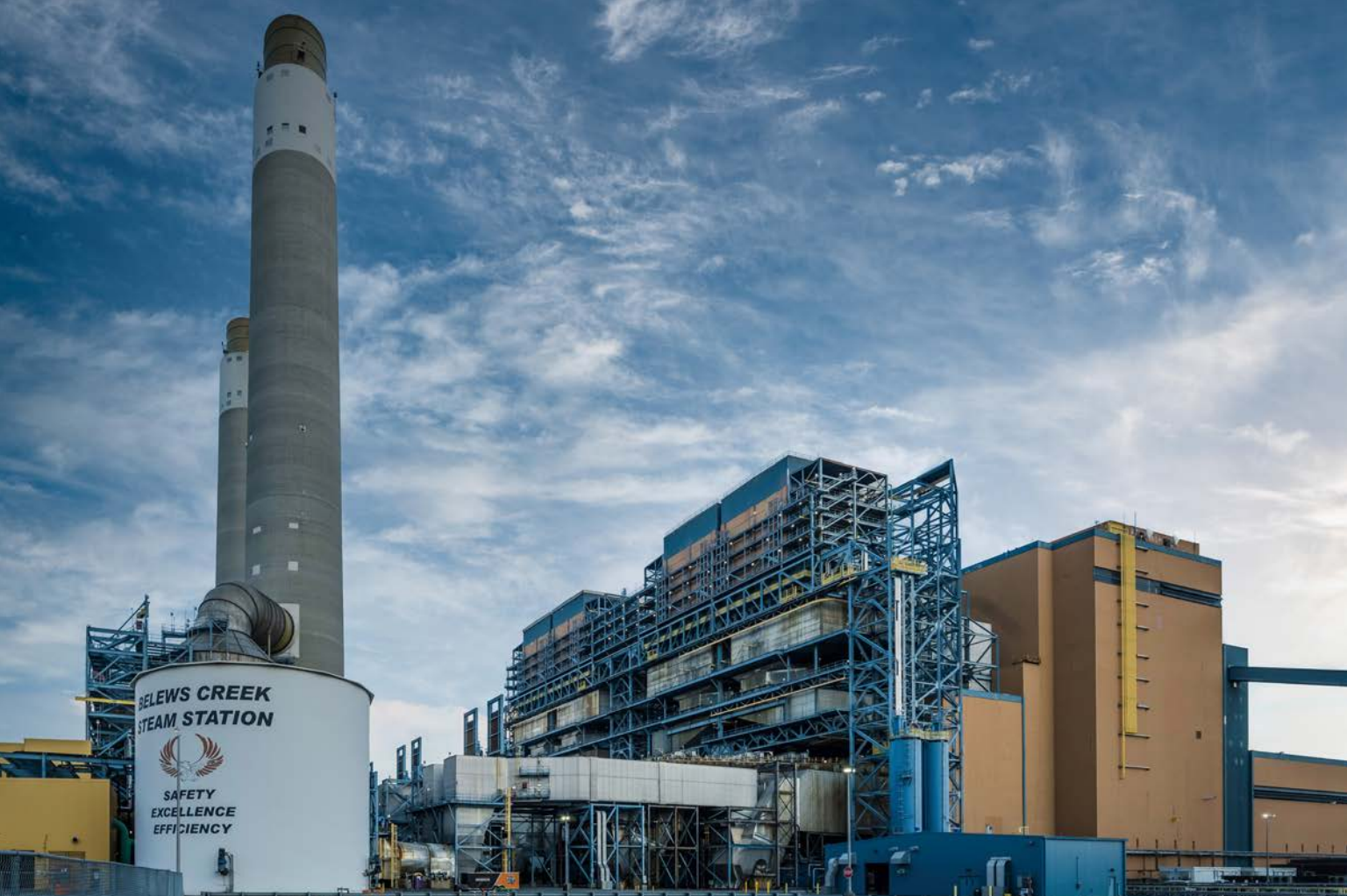
Belews Creek Steam Station
